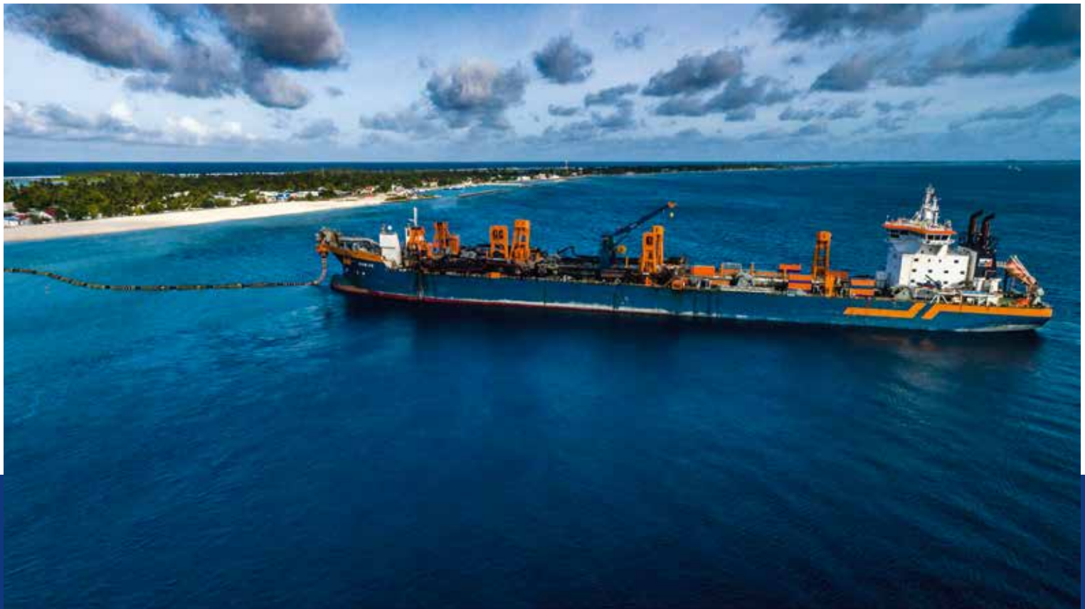
Trailing suction hopper dredger HAM 318 working on the Maldives project
