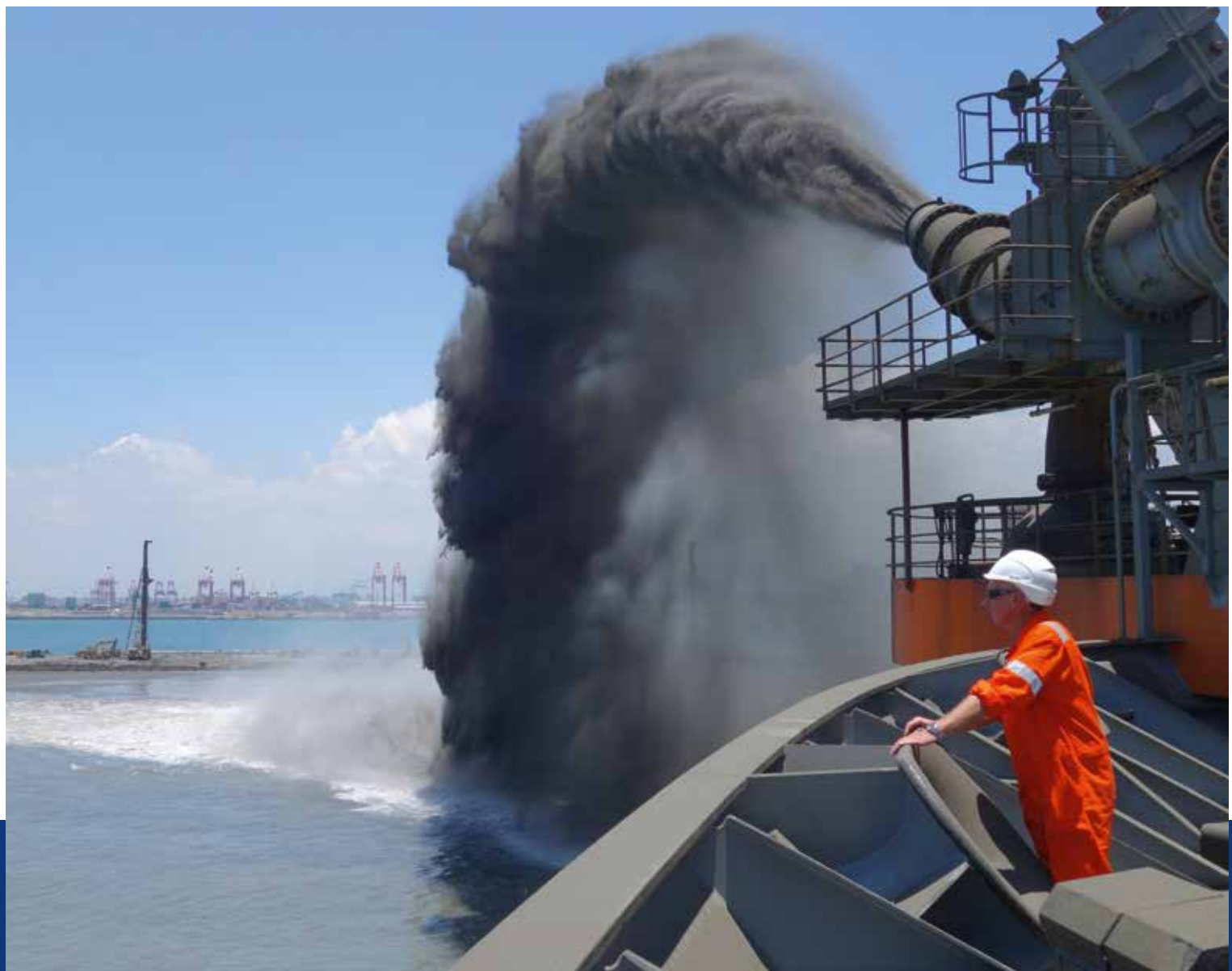
Trailing suction hopper dredger Vox Máxima working on the Kaohsiung land reclamation project in Taiwan
