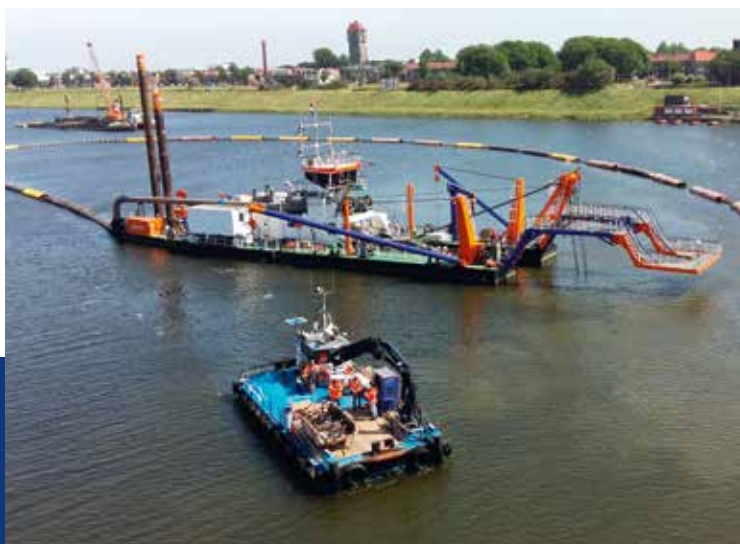
Our new cutter suction dredger Biesbosch at the Sea Lock project in IJmuiden, the Netherlands
