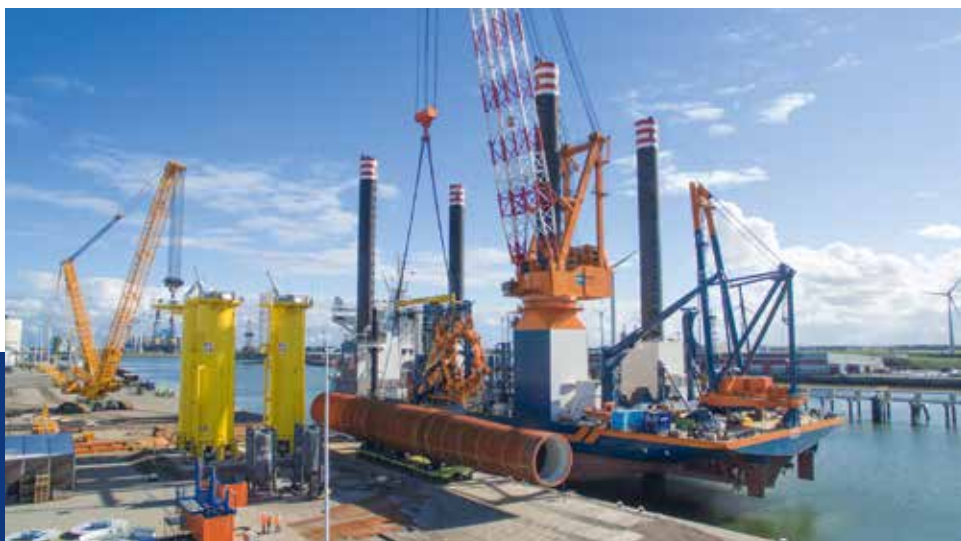
Loading the mono-piles and transition pieces on board offshore installation vessel Aeolus
