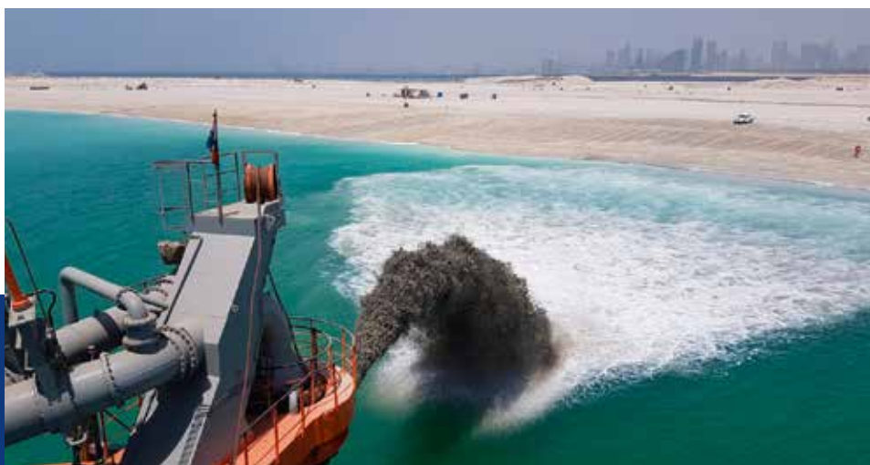
Trailing suction hopper dredger HAM 312 helping to develop the Deira Islands, Dubai
