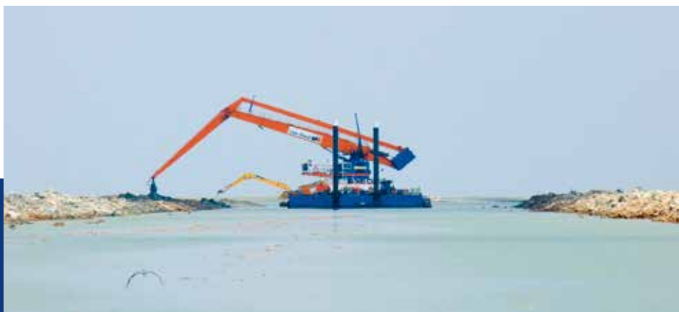
Crane vessel Titan working on the Kashagan project in Kazakhstan
