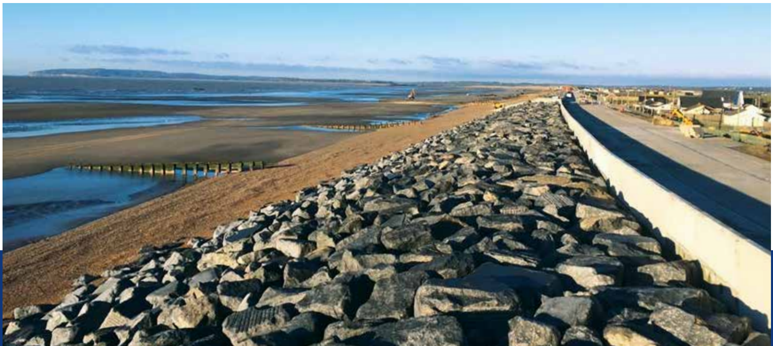
The Broomhill Sands coastal defence project protects against flooding
