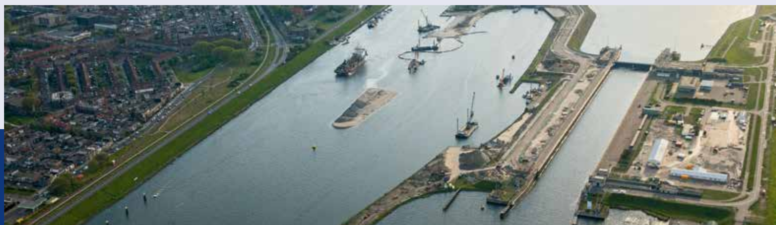
Under construction: new sea lock at IJmuiden
