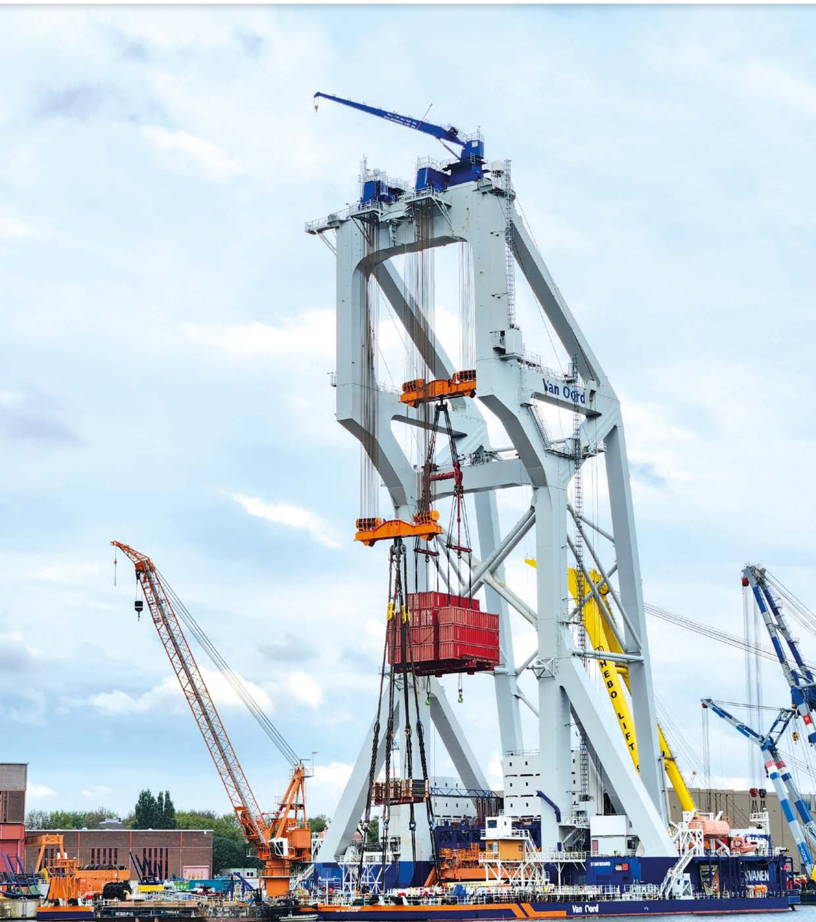
Load test for our upgraded heavy lift installation vessel Svanen. Thanks to the upgrade, including a 25-metre extension of the gantry crane, the Svanen is ready to install the foundations for the next generation of wind turbines.
